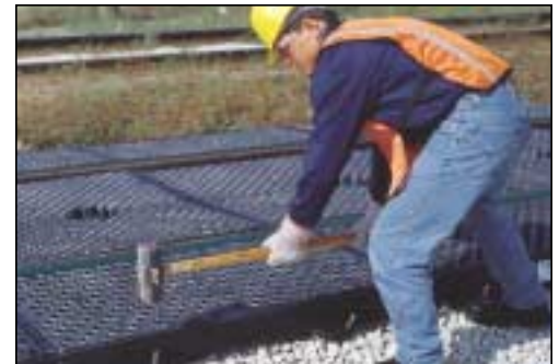
Side Pans are secured in place with rebar or other fasteners. (2-foot-long rebar fasteners with protective caps are available as options.)
