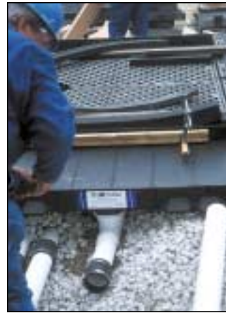
Large, 3"-diameter flow-through channels allow spills to quickly travel from one pan to the next. Channels are located at the low point in each Center and Side TrackPan.
