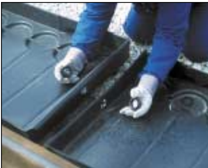
Flow-through channels — All Pans are connected "end-to-end" with bulkhead fittings, and a 3-inch diameter flow-through channel.
