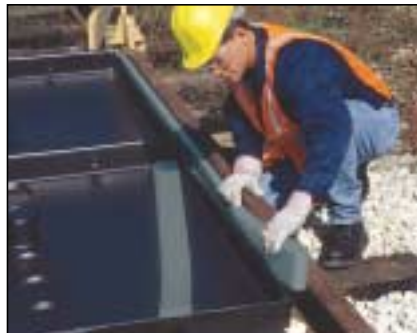
Closed-cell, polyethylene gaskets are then installed to provide a seal between the Pans and rails. (Black gaskets are provided.)
